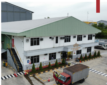
Pergudangan Tembesu 6 No. 1 Tembesu Warehouse 6 No. 1
