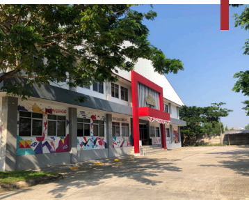
Pergudangan Tembesu No. 7 Tembesu Warehouse No. 7
