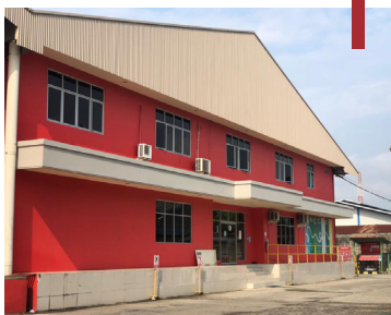
Pergudangan Tembesu 3 No 3 Tembesu Warehouse 3 No. 3
